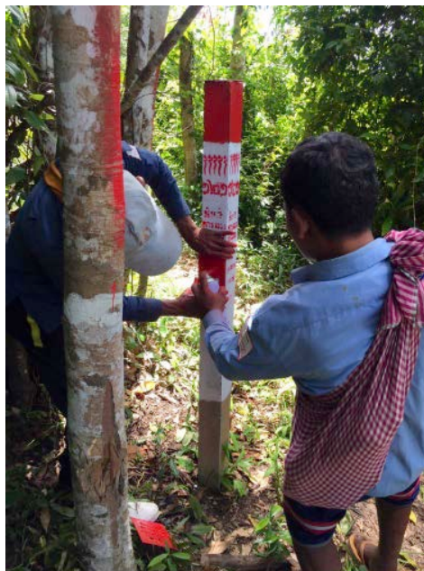
Maintenance of APA cement post, August 2017.
